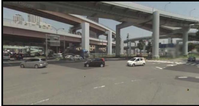
Local Road Underneath
