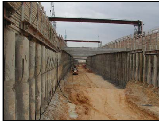
Cut & Cover Tunnel
