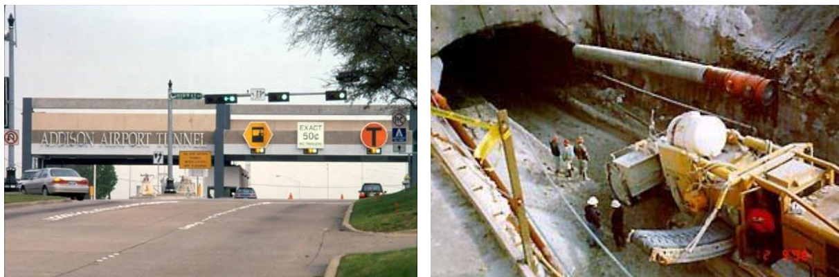
Figures 12/13: Addison Airport Tunnel Entrance and construction
