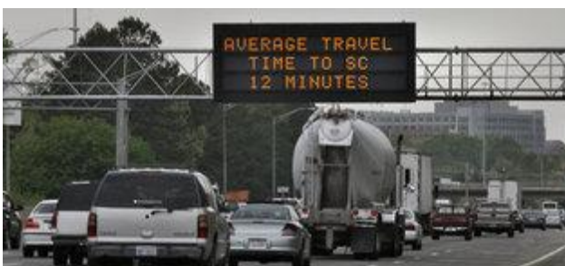
Figure 6: Variable Message Signage
