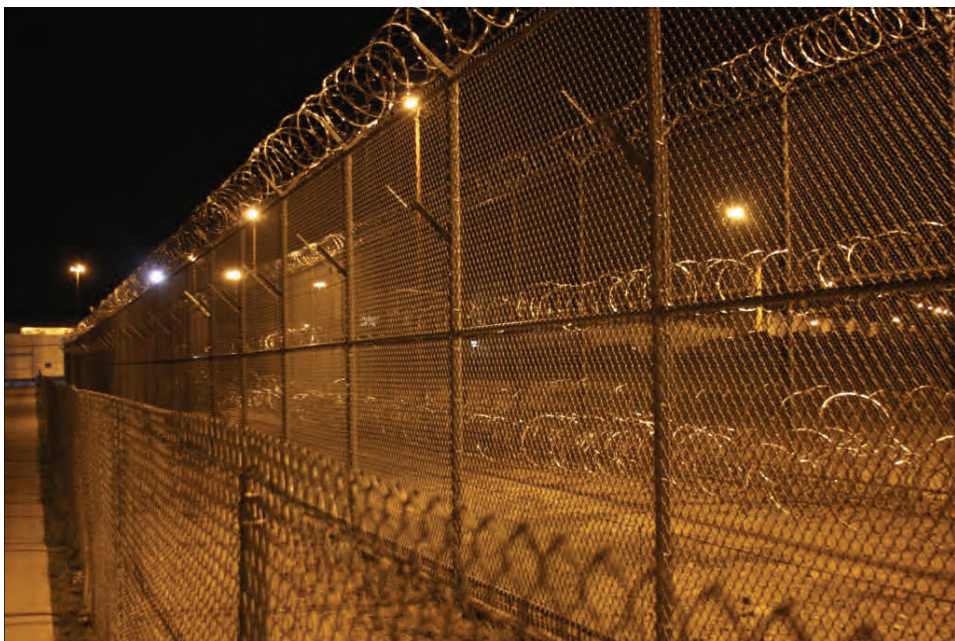
Fencing and razor wire marking the double perimeter of Montana State Prison reflect the glow from high-pressure sodium lights.
