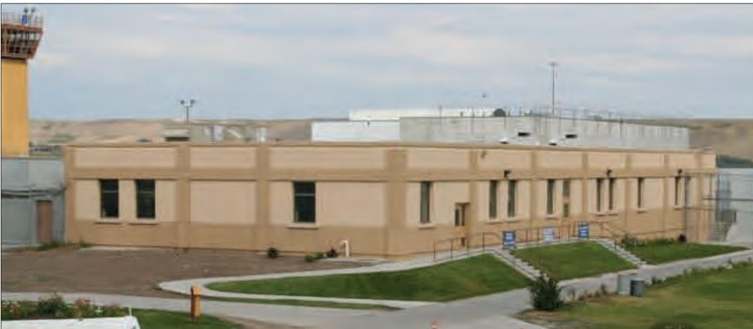
Once an outdated and deteriorating cellblock, this building at Montana State Prison was renovated for use as a visiting room, inmate property office, satellite infirmary and transportation office.
