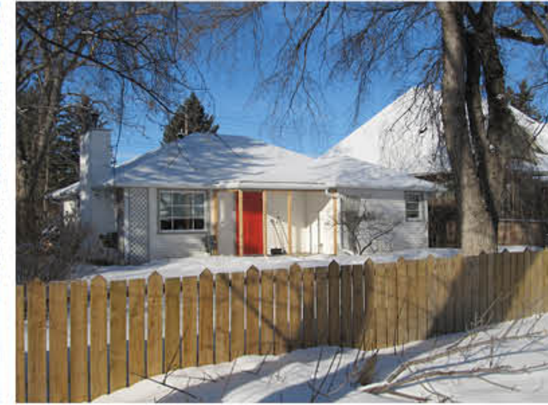
919 - 7th Street Southwest
