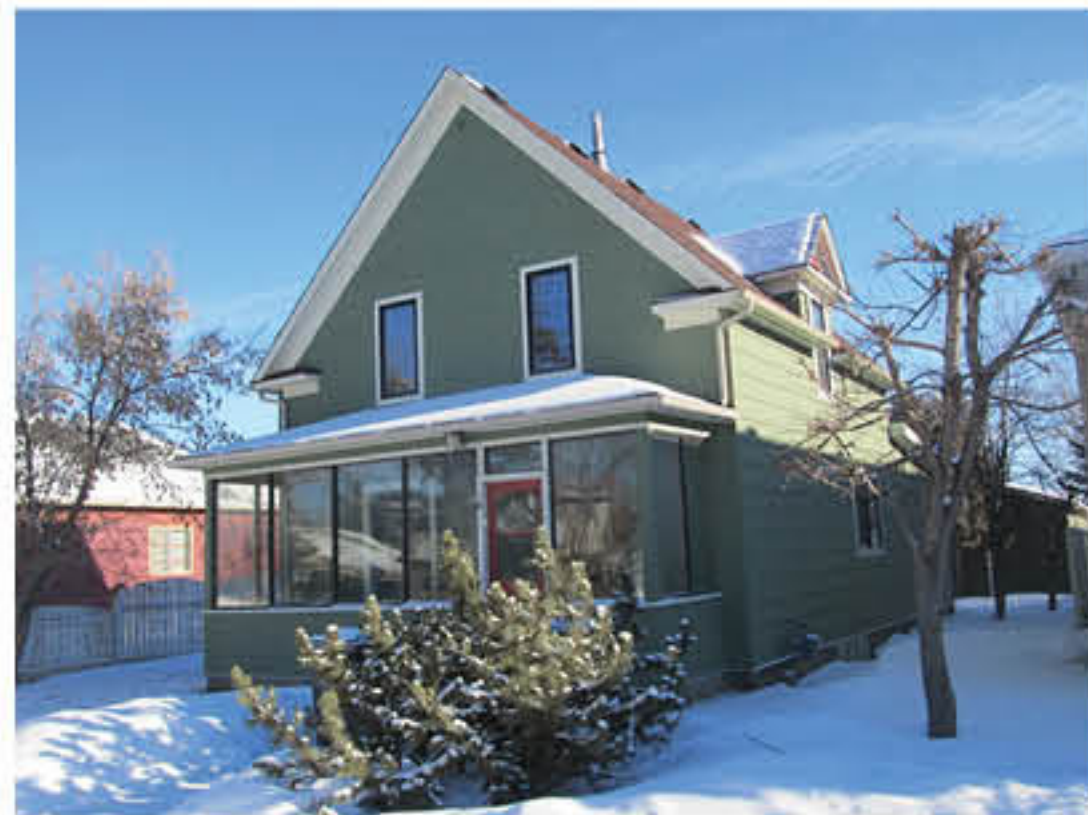
714 - 2nd Street Southwest (1908)
