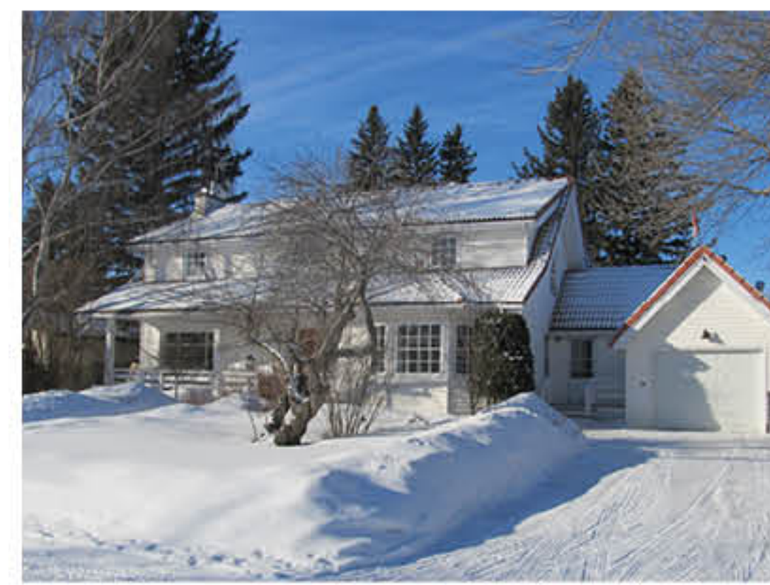
423 - 8th Street Southwest
