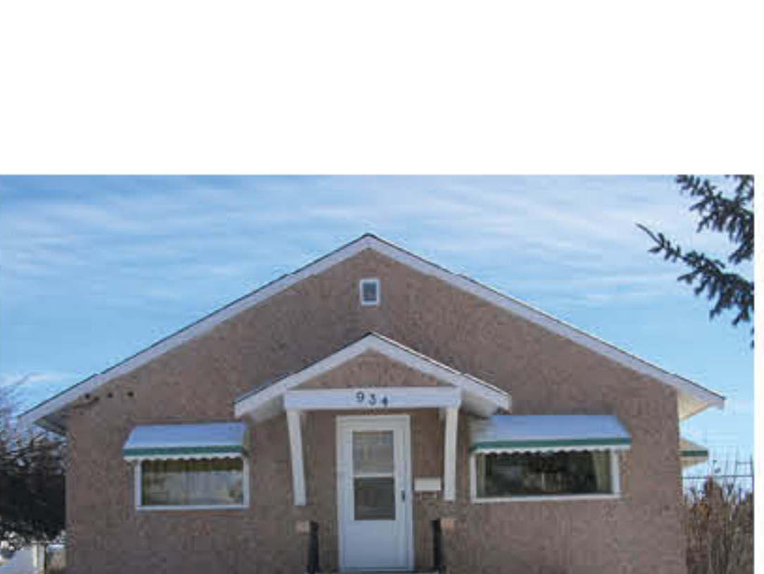
934 - 6th Street Southwest
