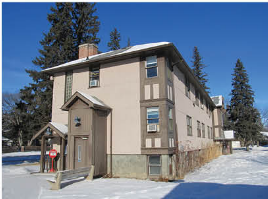
702 - 6th Street Southwest
