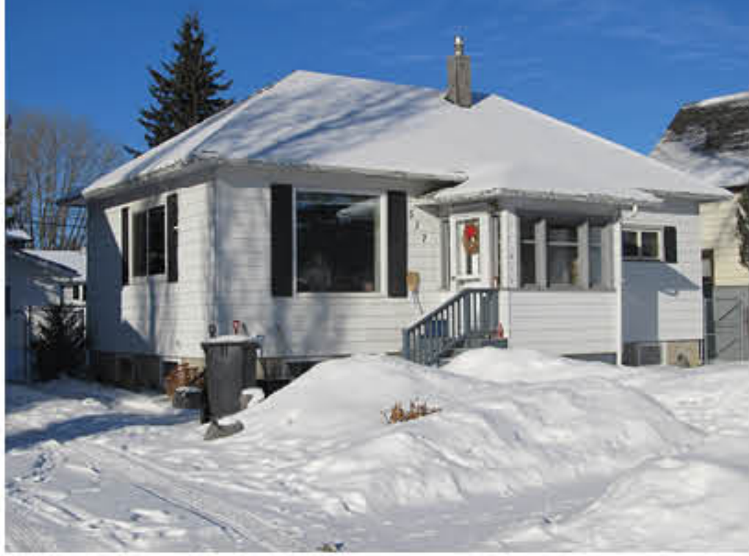
517 - 7th Street Southwest
