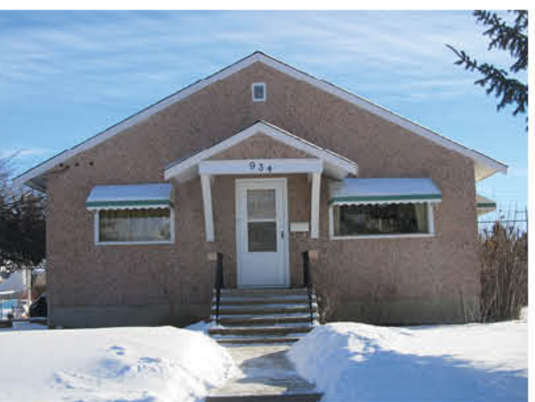
934 - 6th Street Southwest
