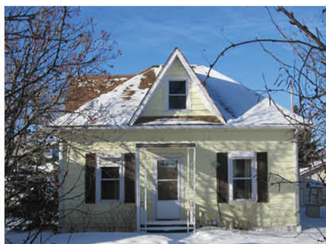
1029 - 6th Street Southwest
