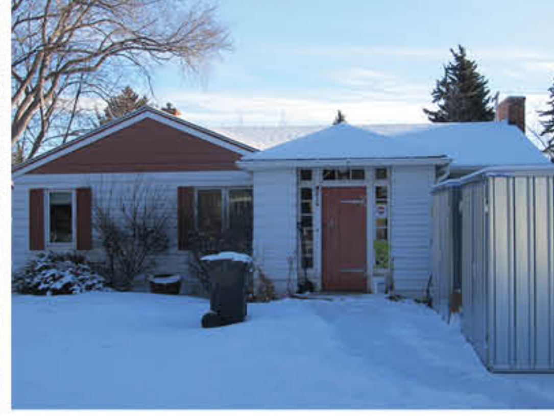
514 - 8th Street Southwest (1950)
