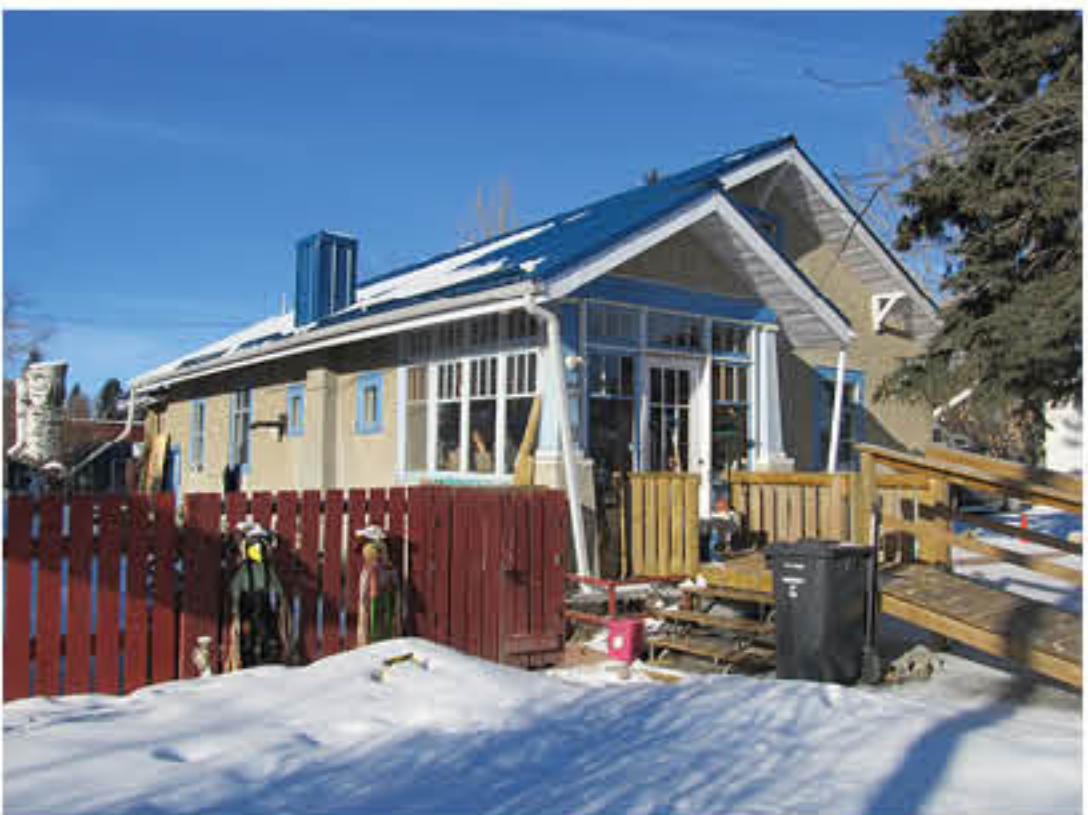
611 - 2nd Street Southwest
