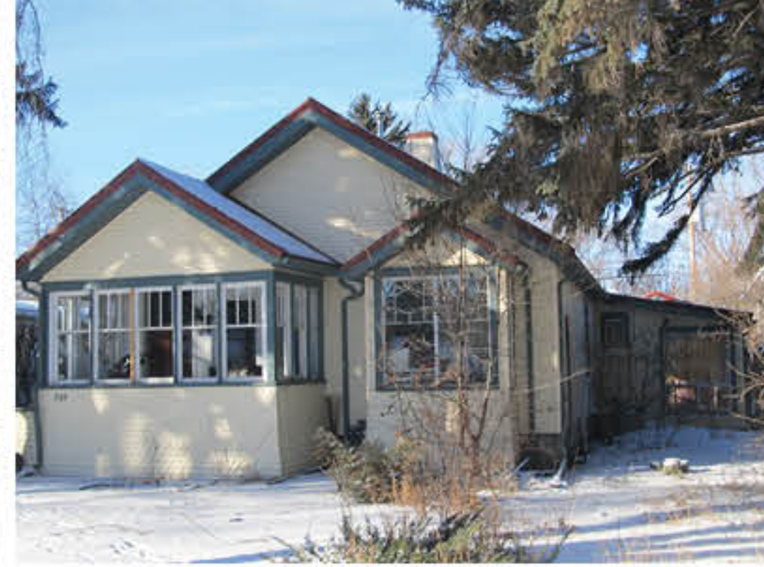
539 - 7th Street Southwest (1910)
