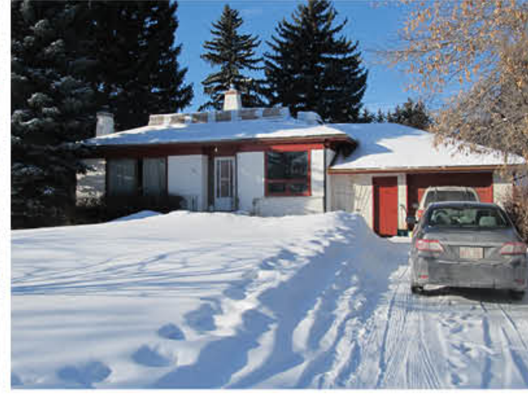
821 - 7th Street Southwest (1946)
