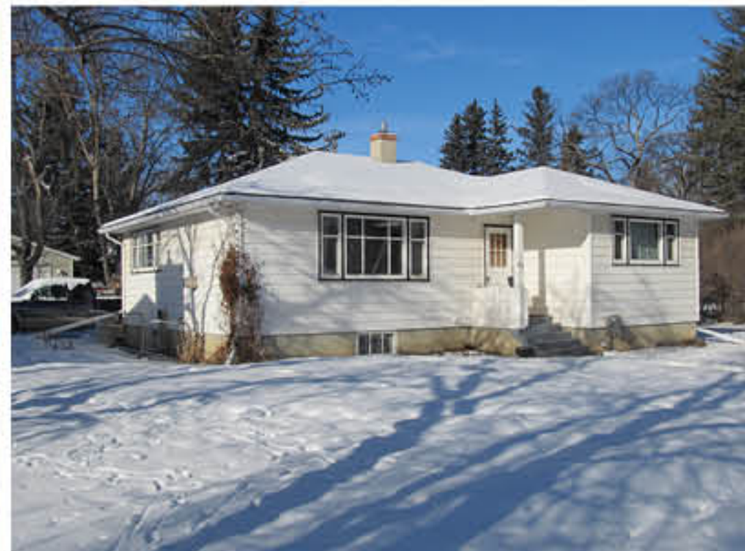
817 - 6th Street Southwest
