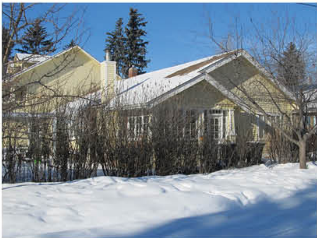
615 - 2nd Street Southwest (1915)
