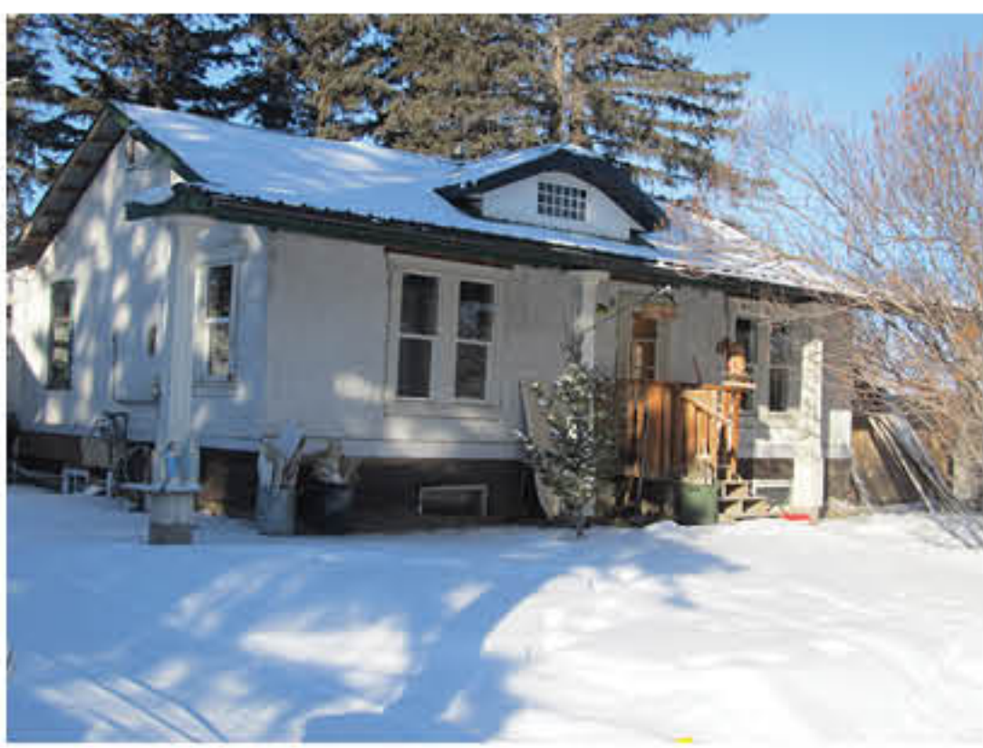
401 - 8th Street Southwest (1949)
