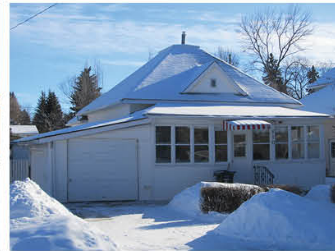
610 - 6th Street Southwest
