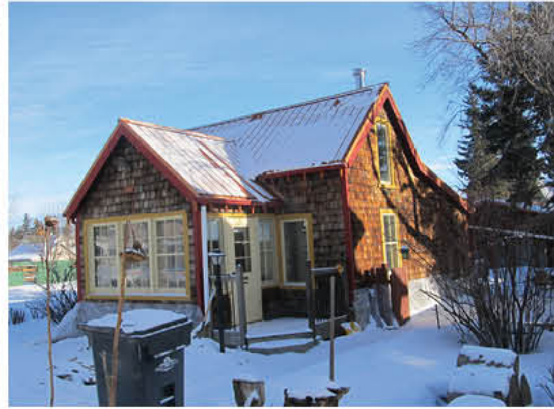
906 - 7th Street Southwest (c1918-36)
