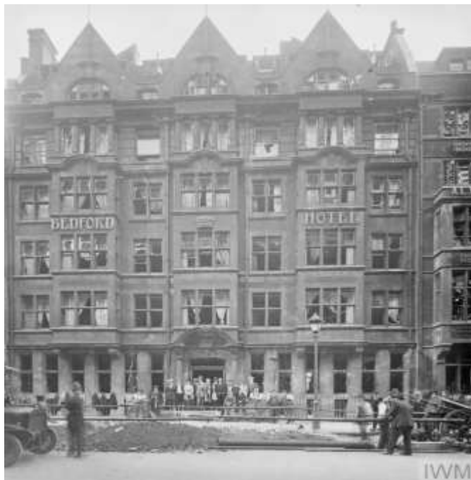
Photo: A group of people stand outside the Bedford Hotel on Southampton Row to watch men at work beside a large crater. The damage was caused by a 50-kilogram bomb during a Gotha raid on the night of 24 - 25 September 1917. The Streamliners were billeted here when they arrived in London around Aug. 20, 1944.
