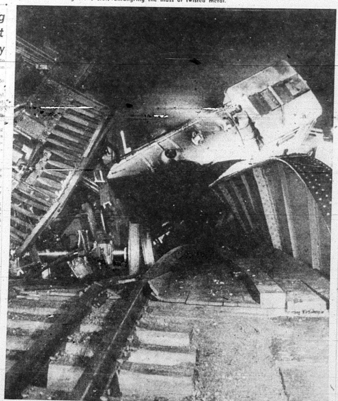
Twisted bridge rail and crushed box cars at scene. (Free Press Staff Photos)
