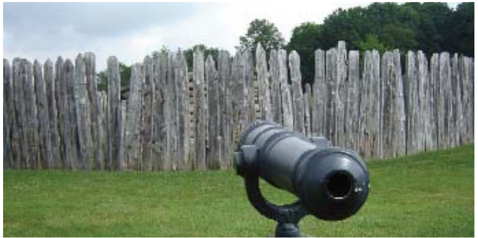
PATHETIC ENGINEERING: A recreation of George Washington’s Fort Necessity sits exposed and vulnerable at the Great Meadows. The National Park Service has kept the tree line to where it was in 1754 when the woods rang with musketry.
