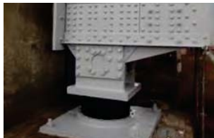
Replaced bearings
