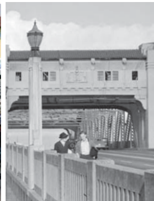
Replace street lighting and allow for future electrical upgrades
