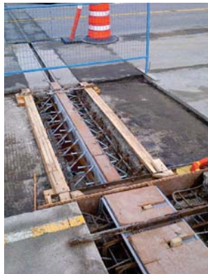
Replaced expansion joints
