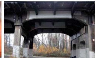
Repaired and strengthened concrete
